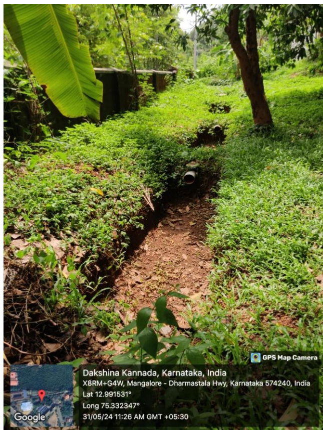
Series of rain water harvesting trenches at SDM College Campus, Ujire
